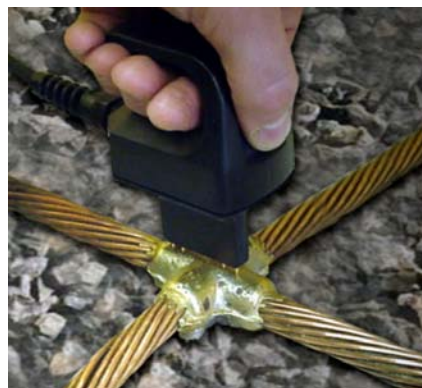
Measuring an aluminothermic joint
