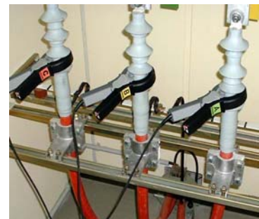
Typical Clamps installation. The clamps can be installed also on cable elbows.
