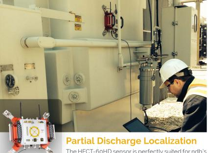
The HFCT-60HD sensor is perfectly suited for ndb's AE-150™ partial discharge localization system for
