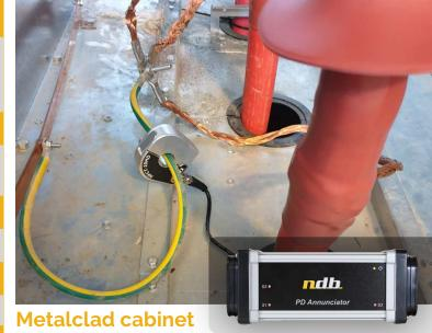
Portable, split-core HFCT sensors are an effective solution for partial discharge measurement and monitoring for metalclad cabinet such as switchgear, ring main unit, cable box, etc.. Pairing ndb's HFCT-HD sensor with the PD Annunciator™ allows for permanent 24/7 partial discharge monitoring with alarm capabilities.
